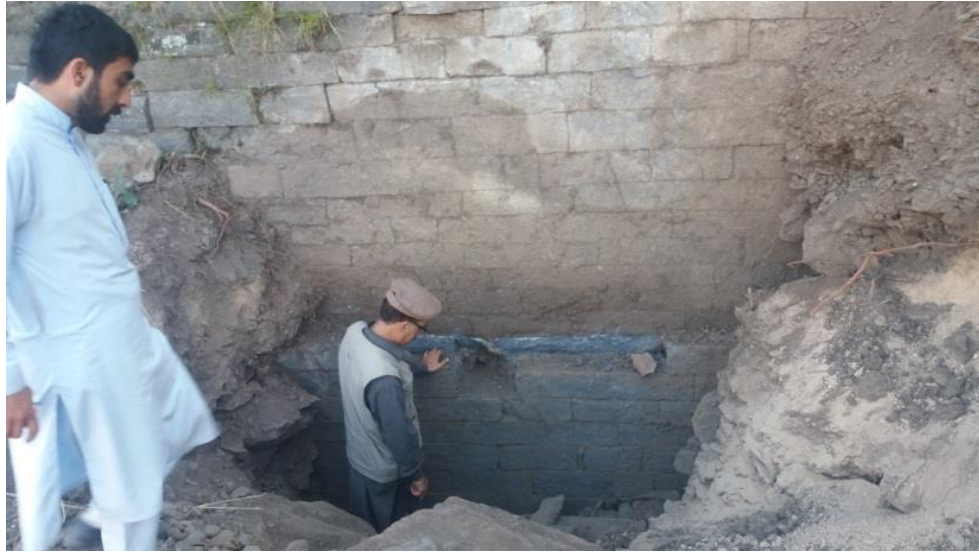
Pl.5. A deep ditch dug by treasure seekers at the foundation of Takht site in Hathi Darah
